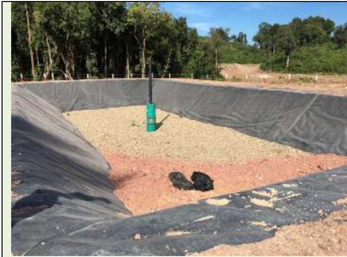
Above: Newly constructed sanitary landfill for the NNP1 project. The landfill is operated by the Main Contractor and supervised by the NNP1PC. Pictures show properly lined disposal cell with impermeable plastic liner and leachate collection system. Cell will receive construction and camp wastes from Contractor and Sub-contractors. These wastes will not contain recovering recyclable materials, which are being removed by all contractors at their camps, prior to transport to the landfill. The photo on the right shows the series of leachate evaporation ponds constructed for long detention time and evaporation of leachate. There are also four observation wells around the landfill to check on groundwater quality and possible contamination from the leachate. NNP1 will manage the site for both and construction and operation phases.
