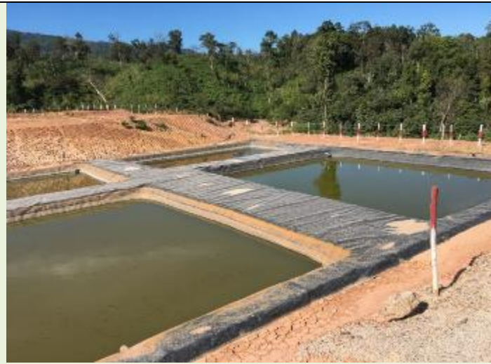
Above: Newly constructed sanitary landfill for the NNP1 project. The landfill is operated by the Main Contractor and supervised by the NNP1PC. Pictures show properly lined disposal cell with impermeable plastic liner and leachate collection system. Cell will receive construction and camp wastes from Contractor and Sub-contractors. These wastes will not contain recovering recyclable materials, which are being removed by all contractors at their camps, prior to transport to the landfill. The photo on the right shows the series of leachate evaporation ponds constructed for long detention time and evaporation of leachate. There are also four observation wells around the landfill to check on groundwater quality and possible contamination from the leachate. NNP1 will manage the site for both and construction and operation phases.
