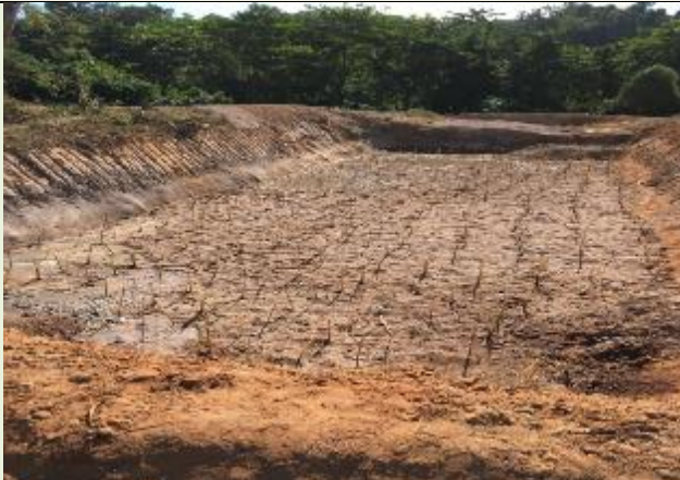
Above: Newly constructed sanitary landfill for the NNP1 project. The landfill is operated by the Main Contractor and supervised by the NNP1PC. Pictures show properly lined disposal cell with impermeable plastic liner and leachate collection system. Cell will receive construction and camp wastes from Contractor and Sub-contractors. These wastes will not contain recovering recyclable materials, which are being removed by all contractors at their camps, prior to transport to the landfill. The photo on the right shows the series of leachate evaporation ponds constructed for long detention time and evaporation of leachate. There are also four observation wells around the landfill to check on groundwater quality and possible contamination from the leachate. NNP1 will manage the site for both and construction and operation phases.
