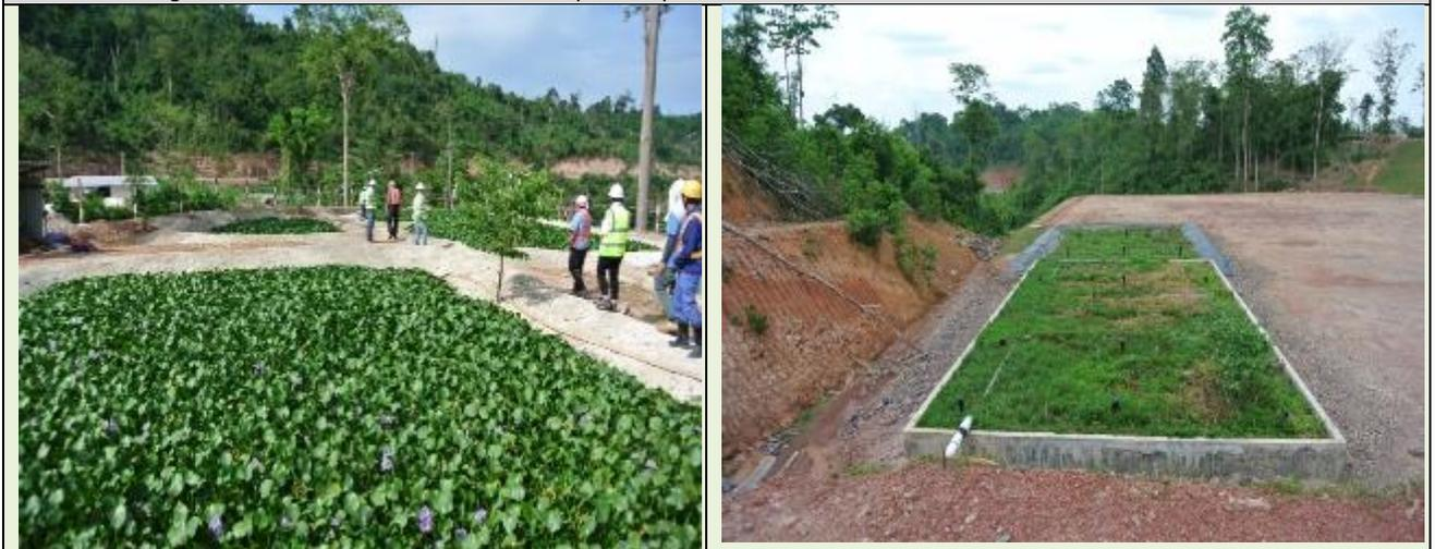
Photo shows improved construction of wastewater pond walls or berms. The ponds have also been replanted with aquatic plants meeting wetlands treatment specifications. However, the effluent still does not meet the Lao Effluent Standards for BOD, COD, and fecal coliforms.
