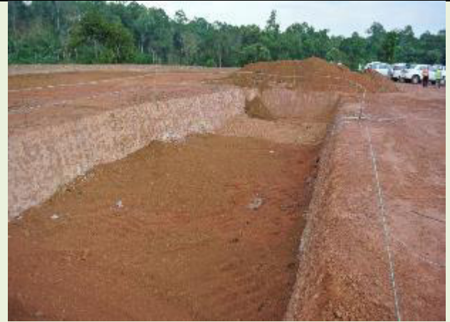
Above: Location of sanitary landfill for the NNP1 project to be operated by the Main Contractor (Obayashi Corp.). Picture shows one “temporary pit” partially filled with construction and camp wastes and covered with a soil layer. These wastes were not separated for recovering recyclable materials. The temporary pits need to be emptied into properly designed and constructed landfill pits, which are double lined with compacted clay and covered with an impervious liner. A leachate collection system needs to be installed and connected to a series of leachate evaporation ponds. The NNP1 Landfill Site should also include a temporary storage facility for separation and storage of recyclable materials, and toxic and hazardous wastes. Obayashi Corp. will manage the site for the entire construction period.
