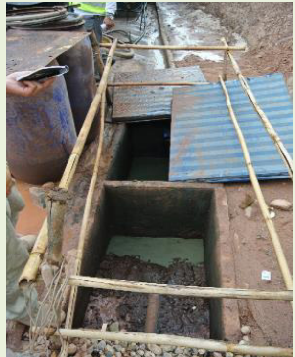
Photo shows the improperly designed and operated oil/grease separator. There is no control valve at the intake. Oil is both drained and washed into the oil separator from an open oil storage area. This area needs the protection bunding and covered roof. Sub-contractor is aware that this facility does not meet environmental safeguard standards.
