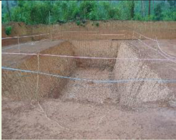
Above: Location of sanitary landfill for the NNP1 project to be operated by the Main Contractor (Obayashi Corp.). Picture shows one “temporary pit” partially filled with construction and camp wastes and covered with a soil layer. These wastes were not separated for recovering recyclable materials. The temporary pits need to be emptied into properly designed and constructed landfill pits, which are double lined with compacted clay and covered with an impervious liner. A leachate collection system needs to be installed and connected to a series of leachate evaporation ponds. The NNP1 Landfill Site should also include a temporary storage facility for separation and storage of recyclable materials, and toxic and hazardous wastes. Obayashi Corp. will manage the site for the entire construction period.
