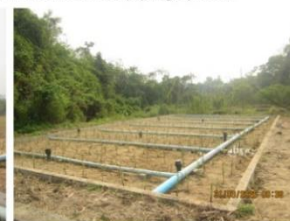
Completed installing new filtration materials, piping system, and planting vegetation
