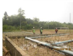
Completed installing new filtration materials, piping system, and planting vegetation
