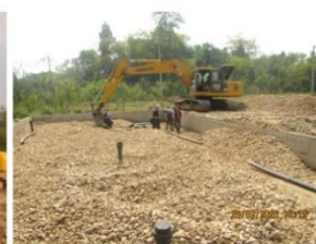
Installed the new filtration materials and piping system
