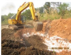
Completed backfilling of wetland vegetation and old filtration sands
