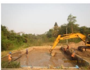
Removal old wetland filtration materials and cleaned up piping system
