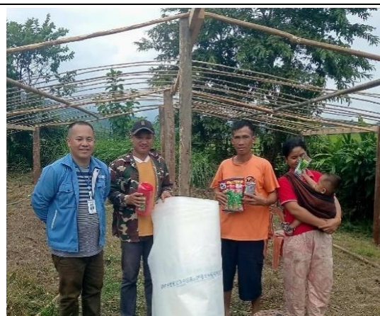
The follow up of greenhouse vegetable construction on 25 September 2024
