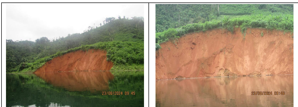
A landslide occurred nearly with the proposed reservoir checkpoint location
