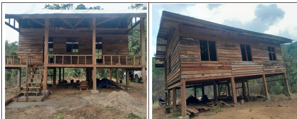
FIGURE 3.2-4 PHOTOS OF NAM SAN PERMANENT SUBSTATION
