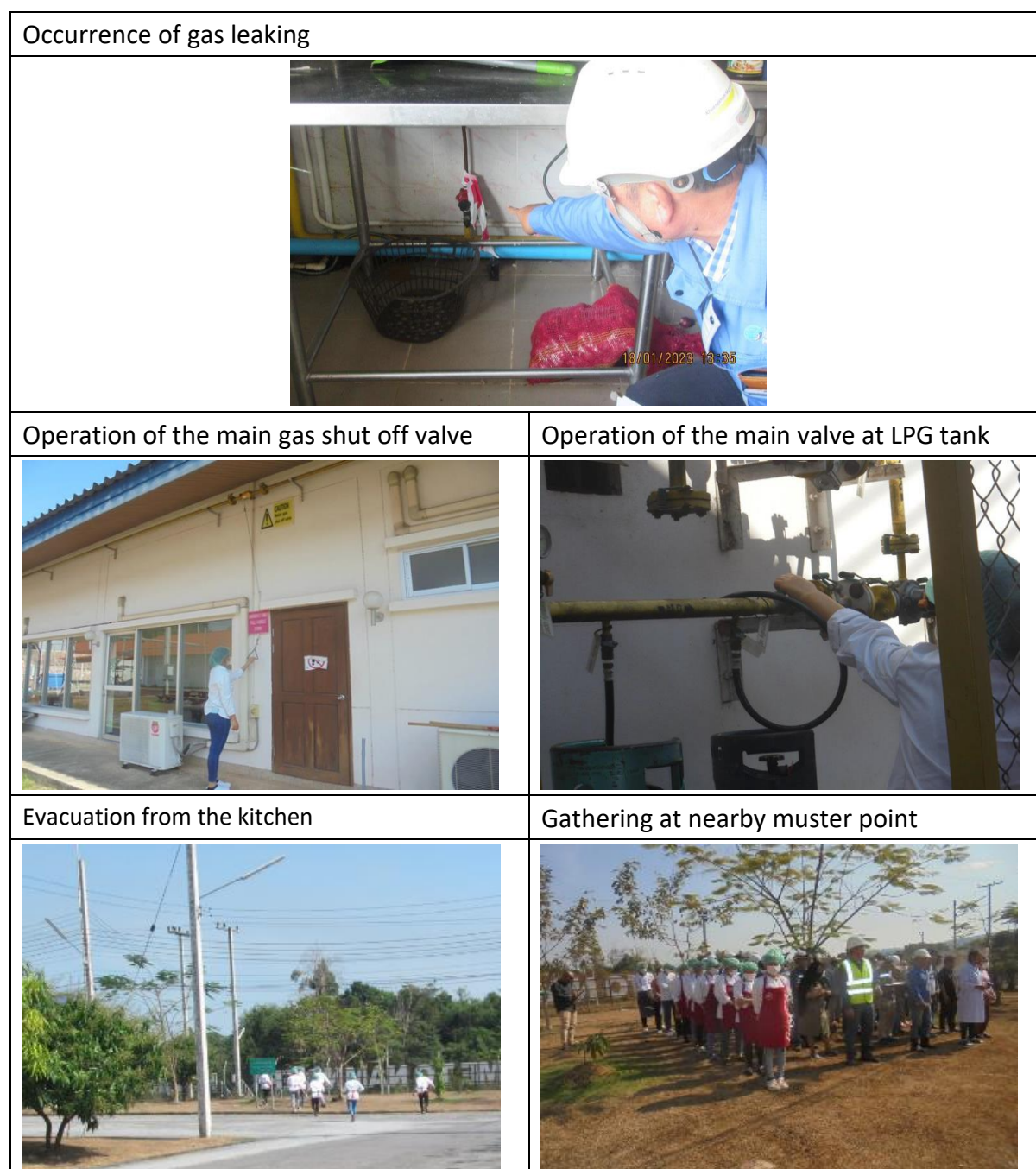
FIGURE 6.1-3. REPRESENTATIVE PHOTOGRAPHS OF CANTEEN LPG GAS LEAK EMERGENCY DRILL
