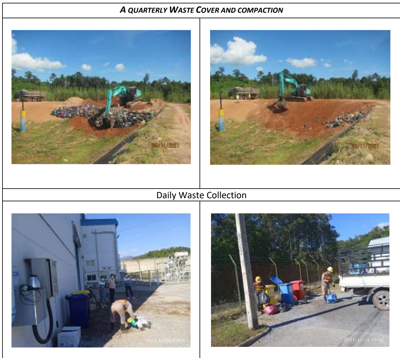
FIGURE 1-7: WASTE MANAGEMENT ACTIVITIES AT NNP1 LANDFILL DURING NOVEMBER 2021
