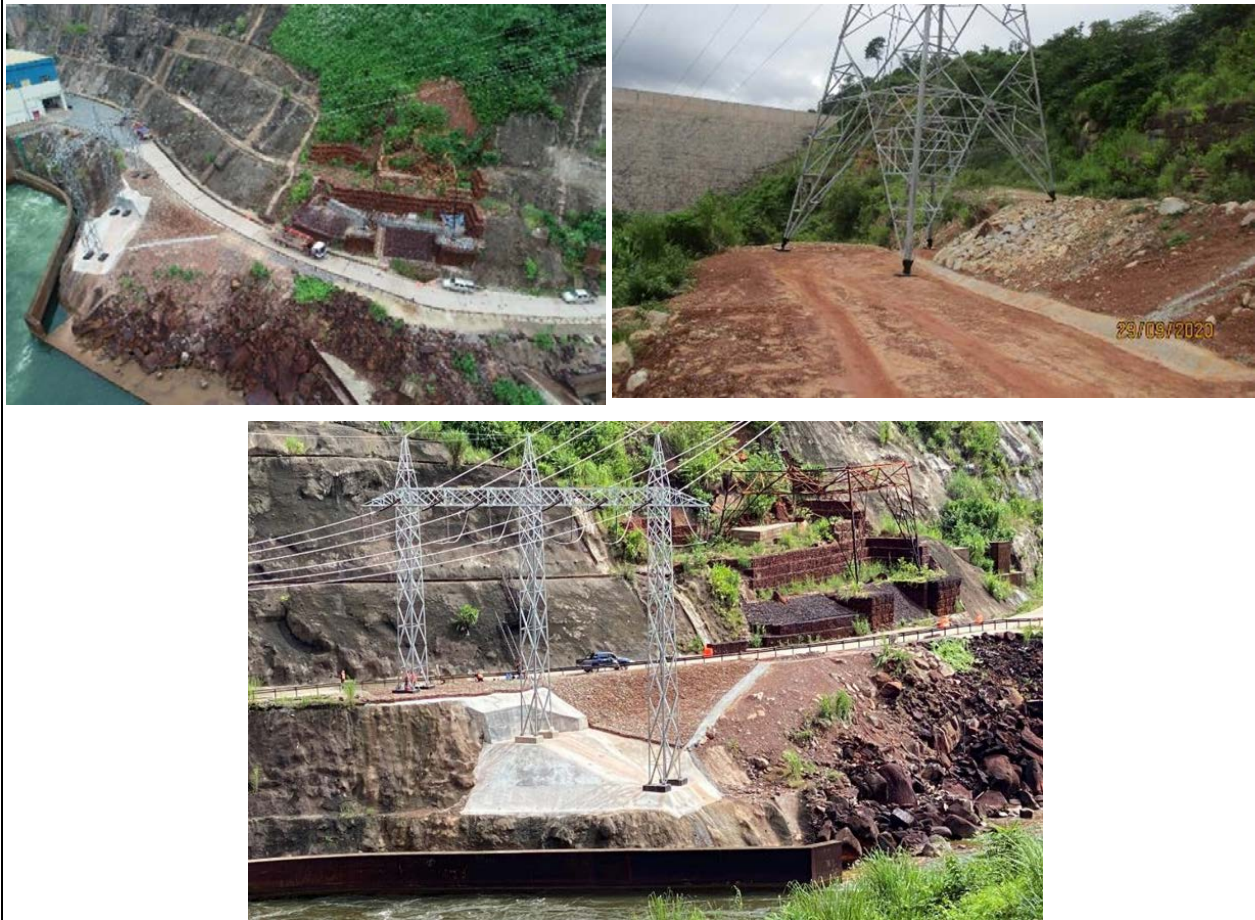
FIGURE 2-14: TOP VIEW OF GANTRY STRUCTURE _SLOPE PROTECTION AROUND FOUNDATION ONGOING
