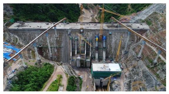
The consolidation drilling and grouting for the main dam started in May 2016 and is ongoing. The progress is 91 % by achievement of total anticipated drilled length as of the end of August 2017 as a proportion of the total expected drilling
