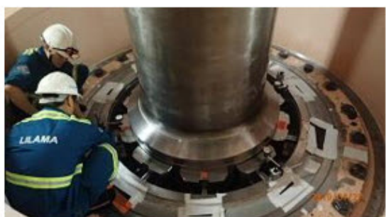
Figure 4.2-3: Assembly of turbine guide bearing for Unit 1
