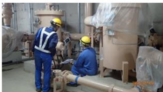
Figure 4.2-9: Operation test of cooling water system for Unit 2
