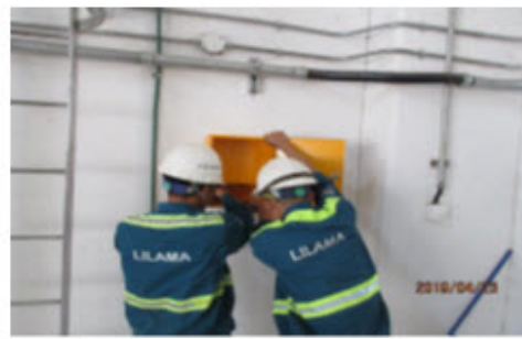
Figure 4.2-14: Punch list work for crane (Installing of remote control box)
