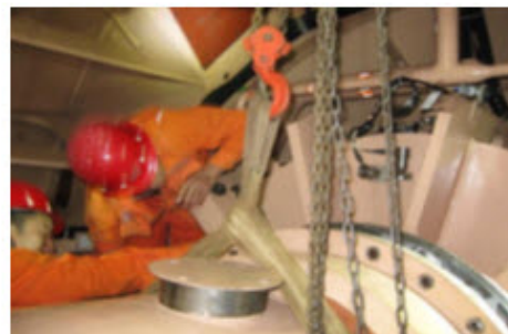
Figure 4.2-12: Punch list work for turbine (Countermeasure for oil leakage)
