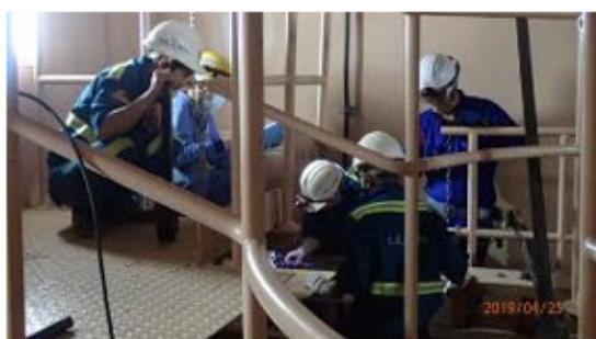
Figure 4.2-8: Adjustment of servomotor arm's position for Unit 2
