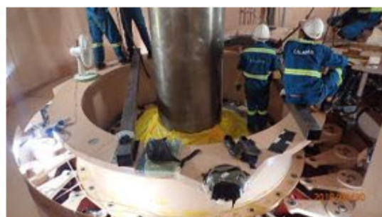
Figure 4.2-4: Assembly of turbine guide bearing cover for Unit 1
