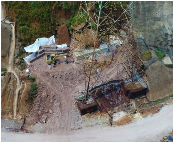
FIGURE 2-8: PREPARATION FOR PLACEMENT OF GABION FOR FOUNDATION BASE OF TOWER NO.1
