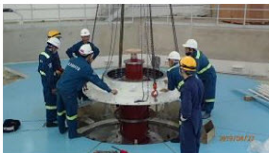
Figure 4.2-1: Assembly of upper guide bearing cover for Unit 1
