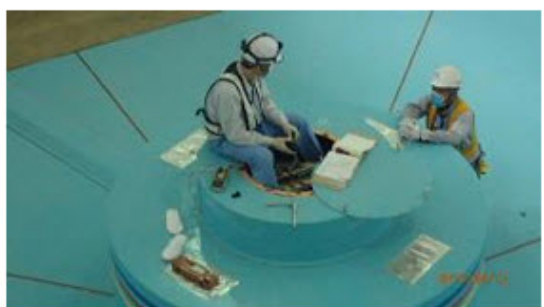
Figure 4.2-5: Wiring connection check of SSG for Unit 2
