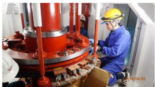
Figure 4.2-6: Assembly of carbon brush of excitation system for Unit 2
