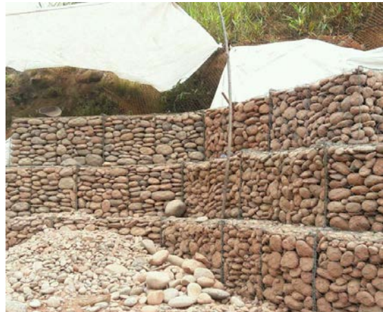
FIGURE 2-8: PREPARATION FOR PLACEMENT OF GABION FOR FOUNDATION BASE OF TOWER NO.1
