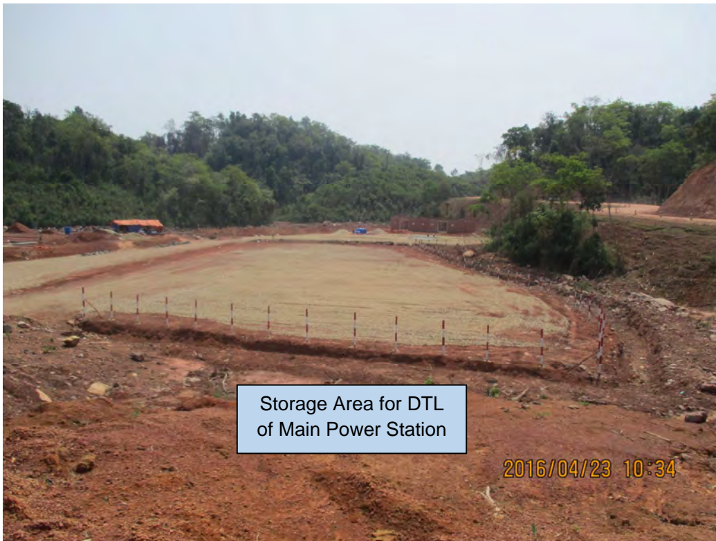
Figure 2-2 Storage yard Area
