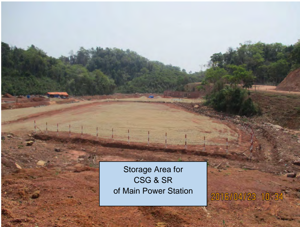
Figure 2-2 Storage yard Area
