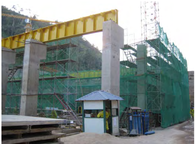
Erection Bay Entrance
