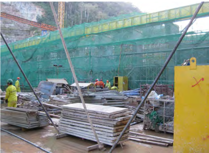
Main Power Station Erection Bay
